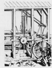
1.4 In the muley saw, variable lengths of the blade could be exposed between the adjustable muley heads. This ability to adapt the saw to the dimensions of logs resulted in a narrower kerf and consequent savings. (Appleton's Cyclopedia, 1880, 2:708.)
