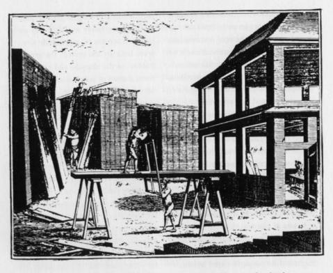
1.2 In this view of an eighteenth-century lumberyard, a frame saw is used to divide a plank laid across trestles. Most of the energy for sawing in this manner was provided by the lower sawyer, and the worker above was responsible for guiding the cut along a chalked line. (Diderot, Encyclopedie, 1762–1777, "Menuiserie," plate 1.)
