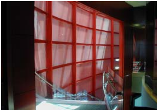
Reginald F. Lewis Museum, Stair and Screen Wall Perforated metal sheets allow transparency and catch the light.
